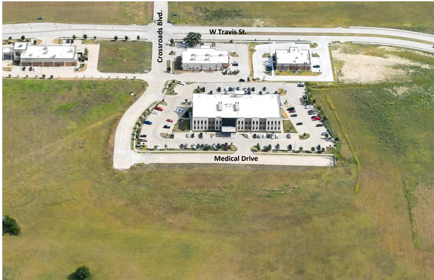
Completed MOB, DaVita, ER and Imaging Center
